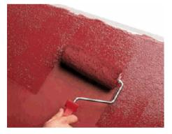
6 Before painting commences prepare a plan of how the tins of paint are to be distributed over the surface. Separate the area to be painted into reasonable sections and distribute the paint tins accordingly. This method helps to achieve a more even distribution of paint over the entire surface and ensures the quantity of paint corresponds to the specification.
