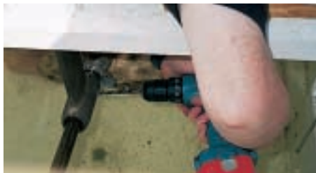
With a battery-powered drill, you can even fit a cutter between tides on a drying mooring
